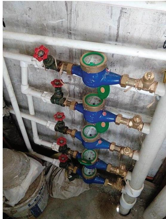
Fig. 4. Domestic Water Meter Accuracy
